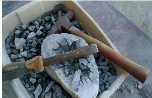
Hammer and chisel out the cut pieces
